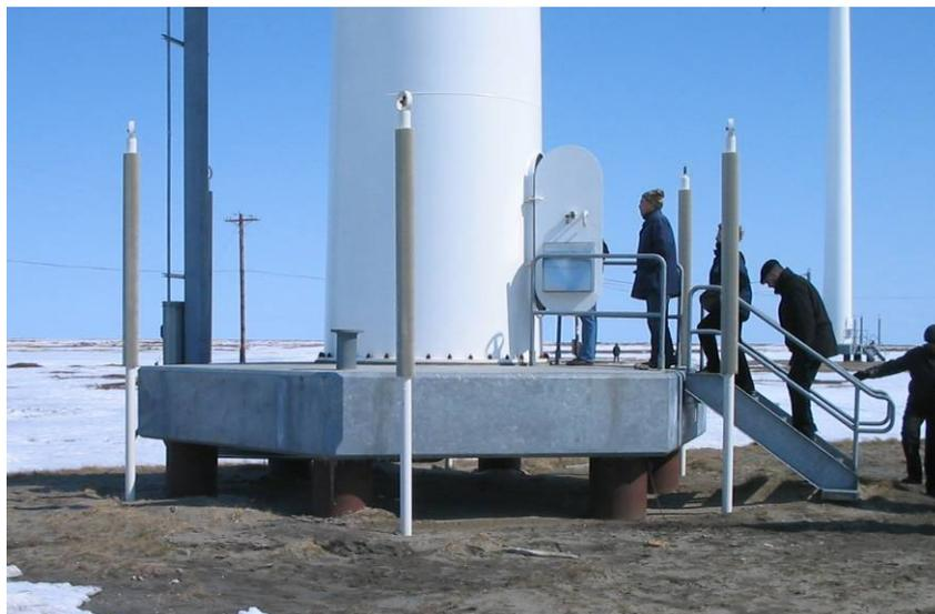
Figure 12. Permafrost foundation for a 100 kW wind turbine in Alaska using thermo siphons and freeze back peers driven into the permanently frozen layers. Photo credit Ian Baring-Gould.
