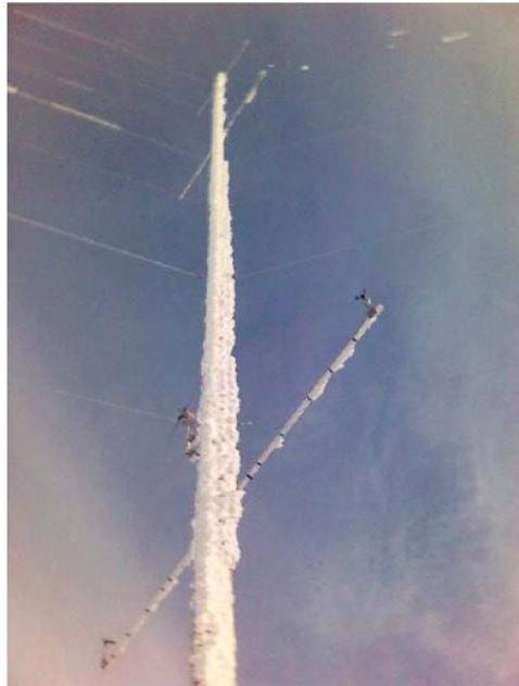
Figure 3. Meteorological tower with heavy icing.
