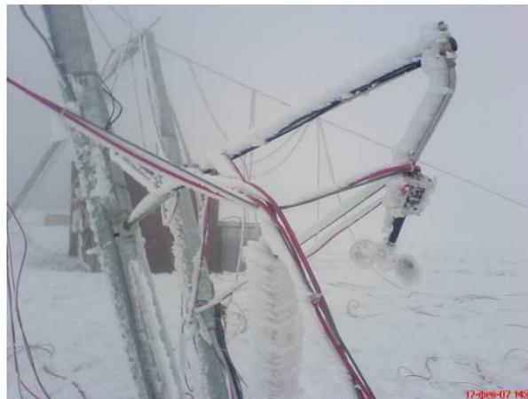
Figure 4. Collapsed meteorological tower, likely due to heavy icing.
